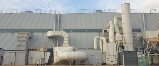
Heat Exchanger for Waste Heat Recycling at the Gunsan Plant
